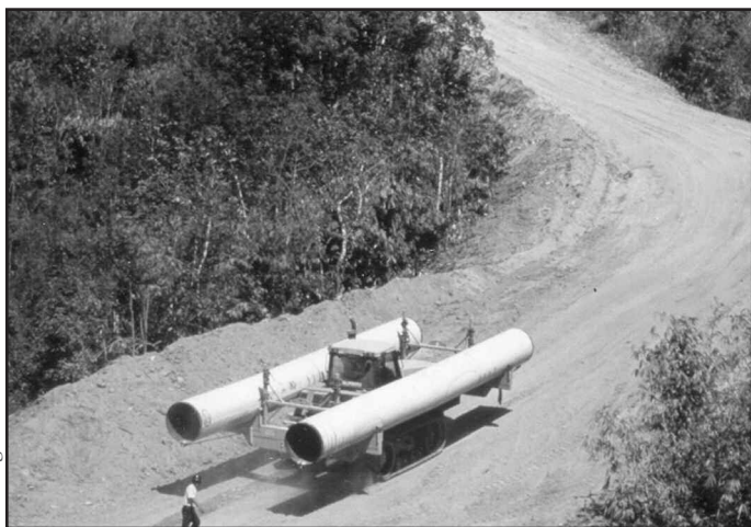
Workers assemble the Yadana gas pipeline.
