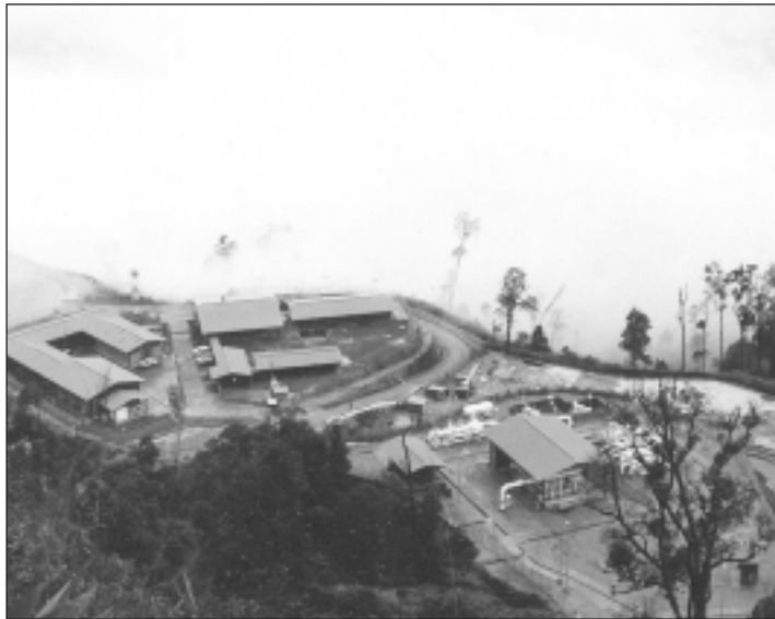
Helipad used to facilitate the construction of the Yadana pipeline.
